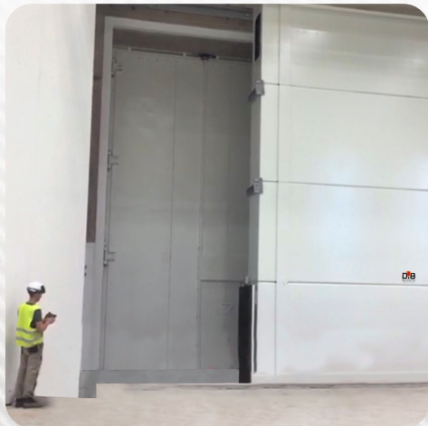
Porte blindée lourde Rolls Royce 380 tonnes - 12m*10m*1m
